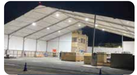
Aircraft Maintenance Hangar
